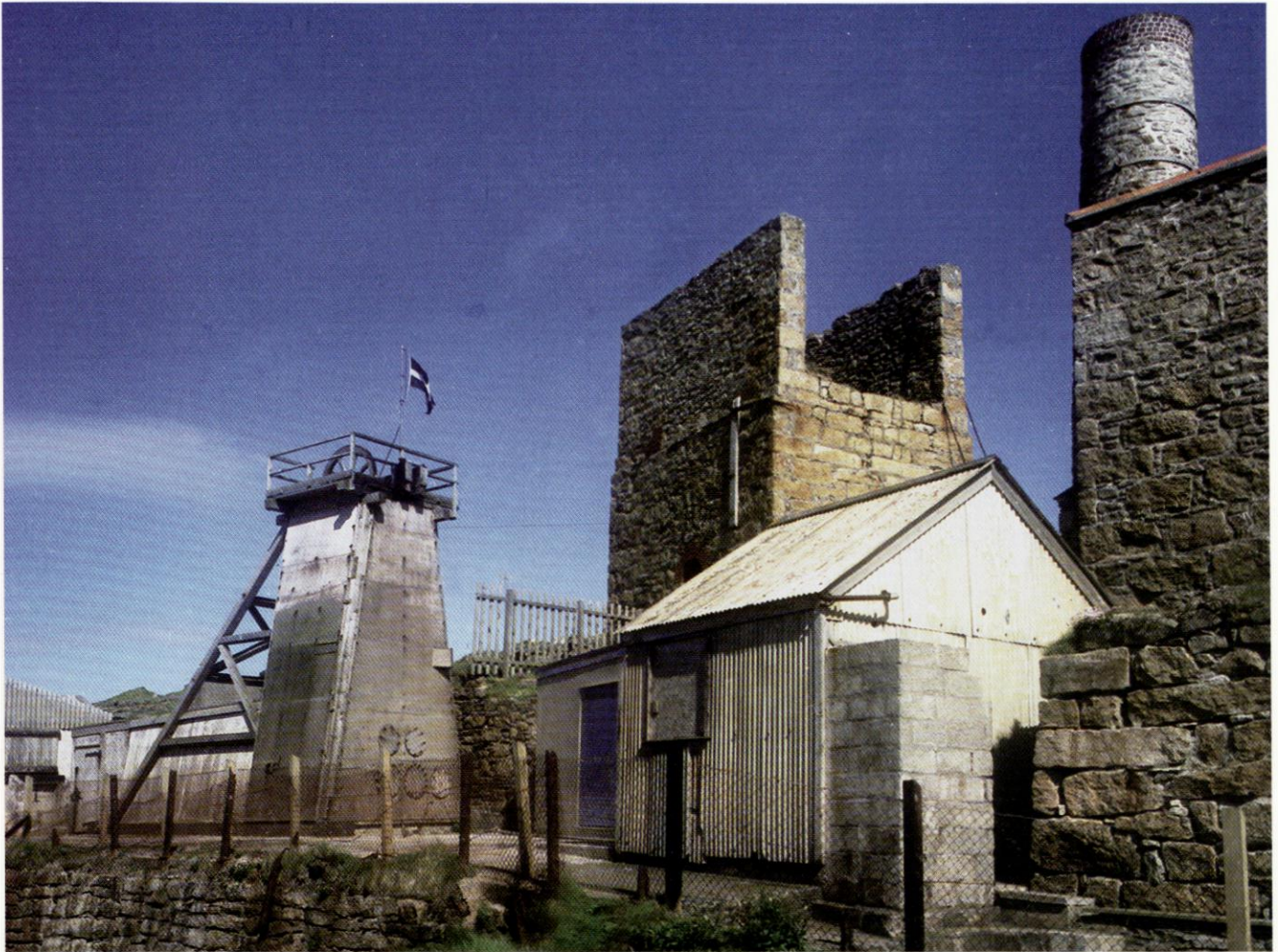
Levant Mine in May 1995. Photo: Nick Catford
